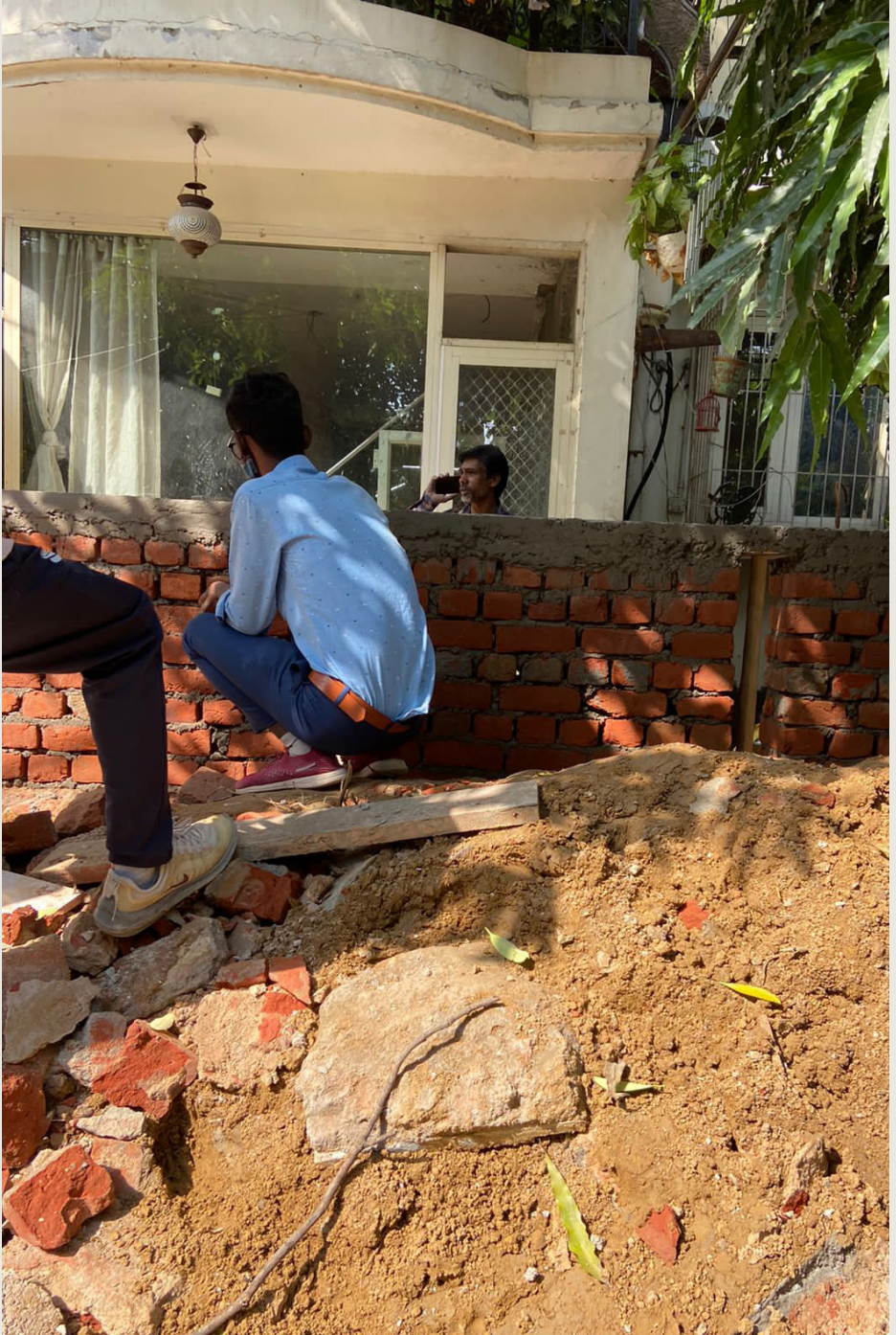
Demolishing - Construction Waste
