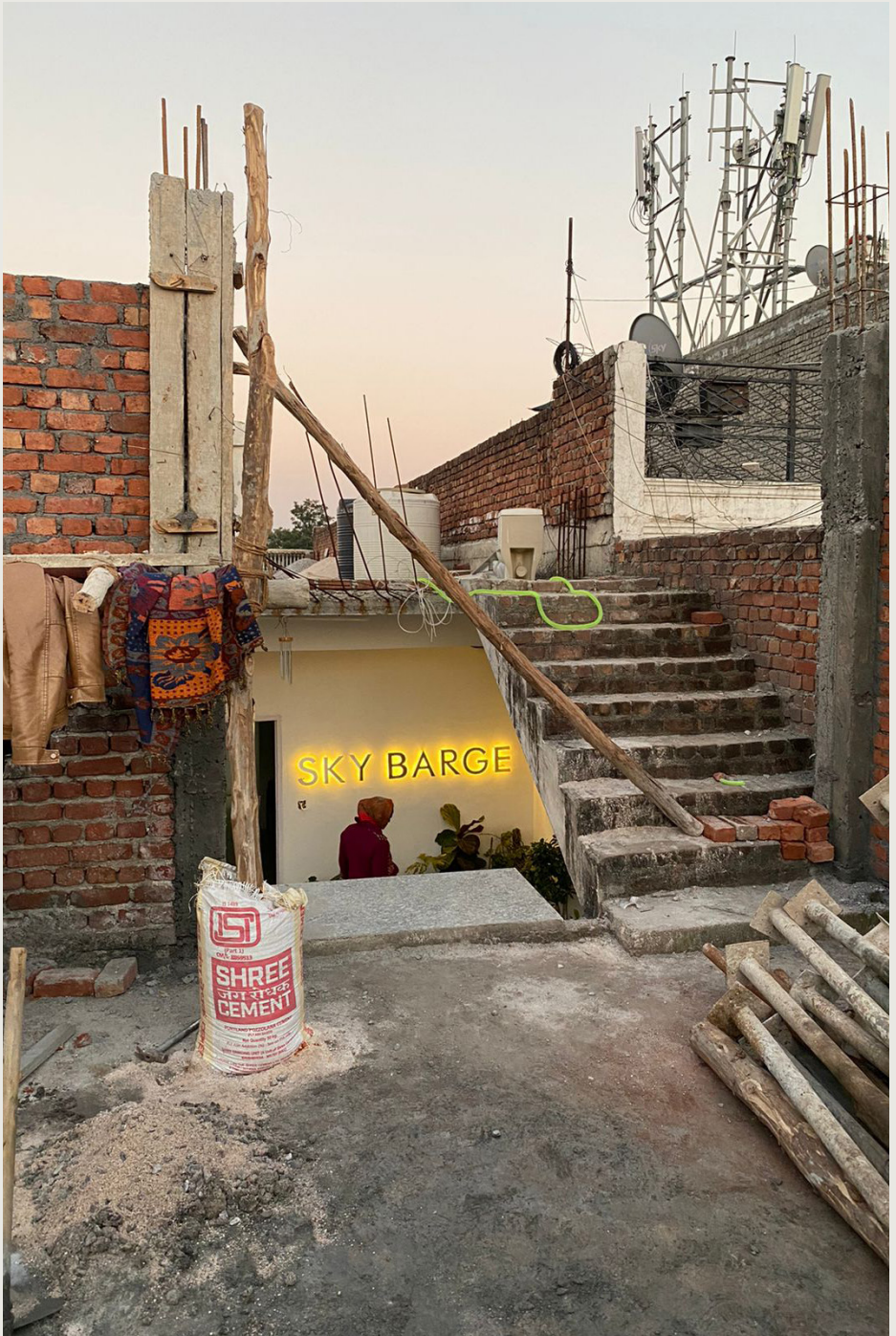
VIEW FROM THE NEW OFFICE - BEFORE
